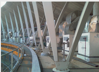
Vulcano Buono – View of 42 rooftop and one of the heat pumps for the shops
